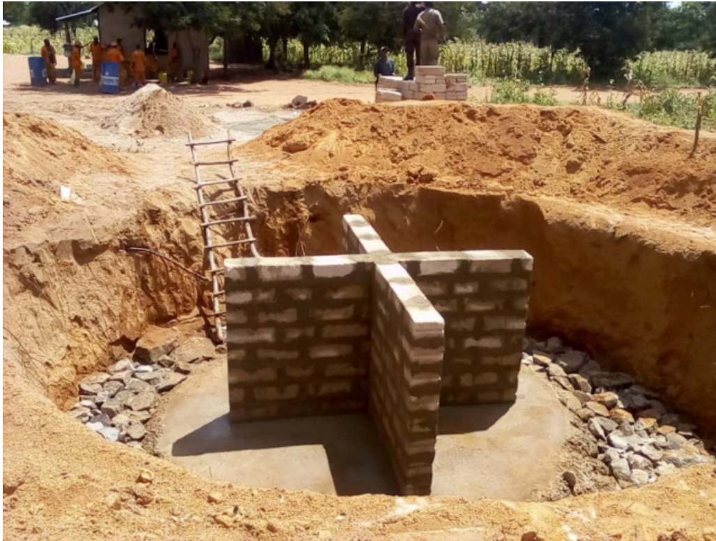
2019 05 14 Construction of tank foundations
